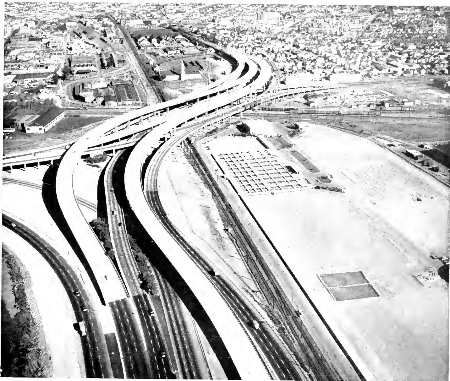
View looking easterly, showing East Bay distribution structure as reconstructed
